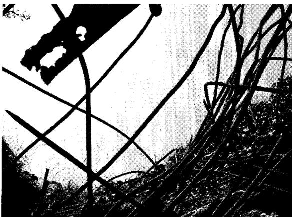
Fig. 10. Bomb impact on concrete roof.
